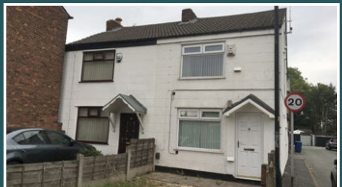
Photo 1: Auction purchase with no space to insulate solid masonry gable wall
