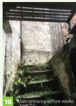
10 Main entrance before works
