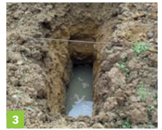
3 External groundwater level visible in trial pit
