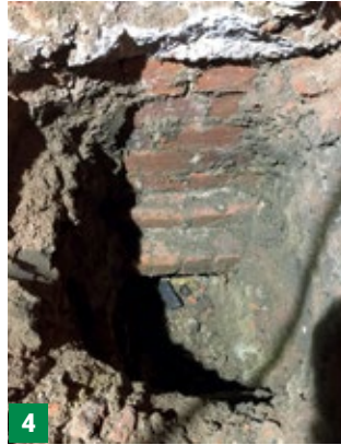
4 Internal trial pit
