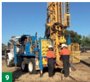
Rotary drilling rig
