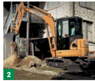
2 Backhoe excavator for external trial holes
